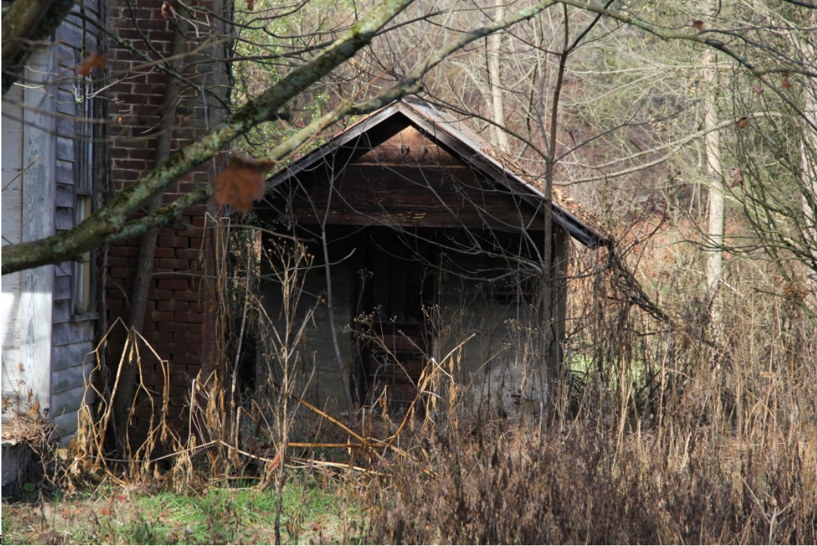
Spring house, facade, view to northwest
