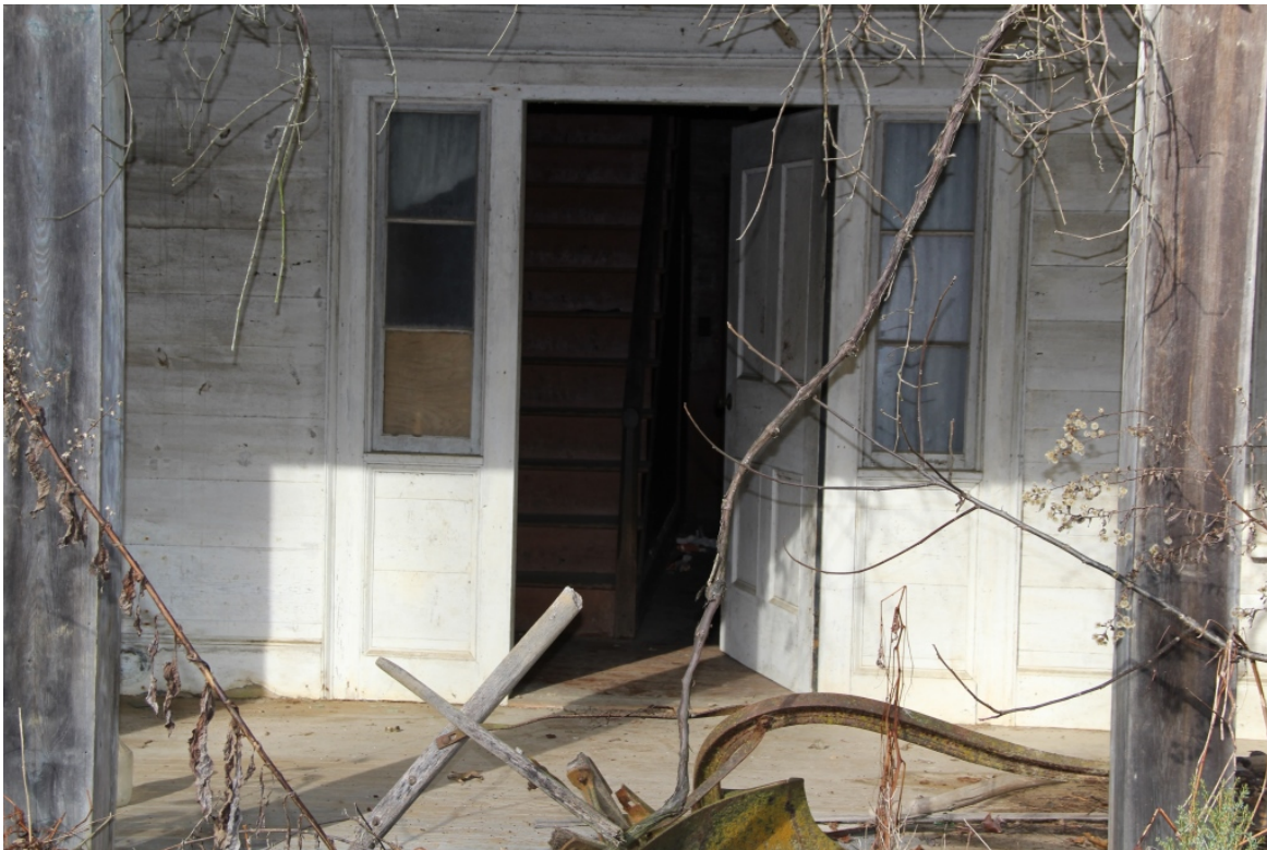
John W. Wells House, entrance detail, view to northwest
