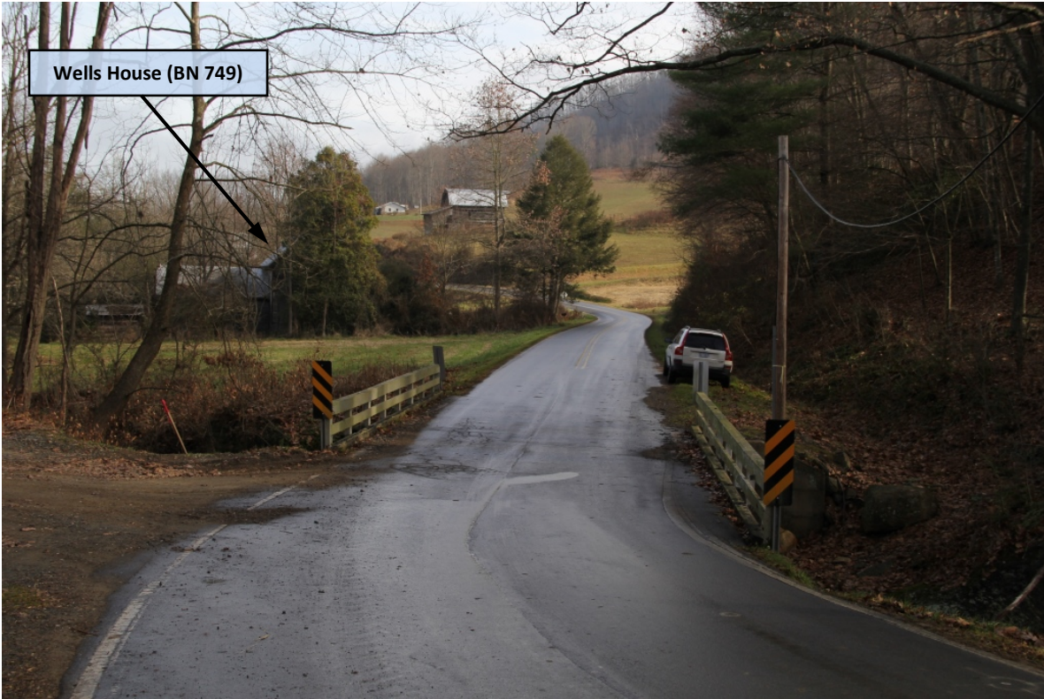
Bridge No. 371 on SR 1394 (Willow Creek Road) over Willow Creek, view to northeast
