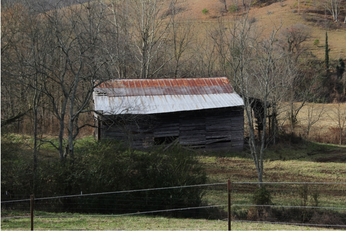
Large barn, side elevation, view to southwest
