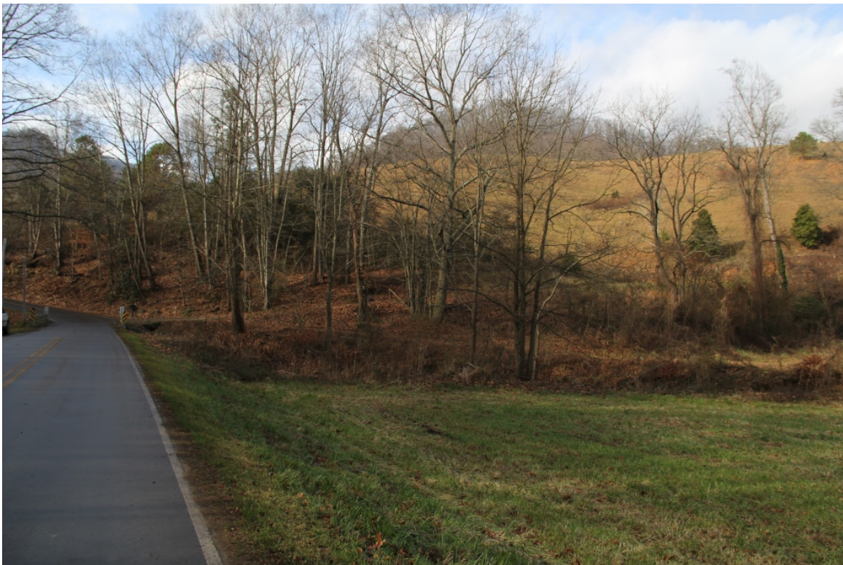
View to southwest along Willow Creek Road (SR 1394); Bridge No. 371 at left
