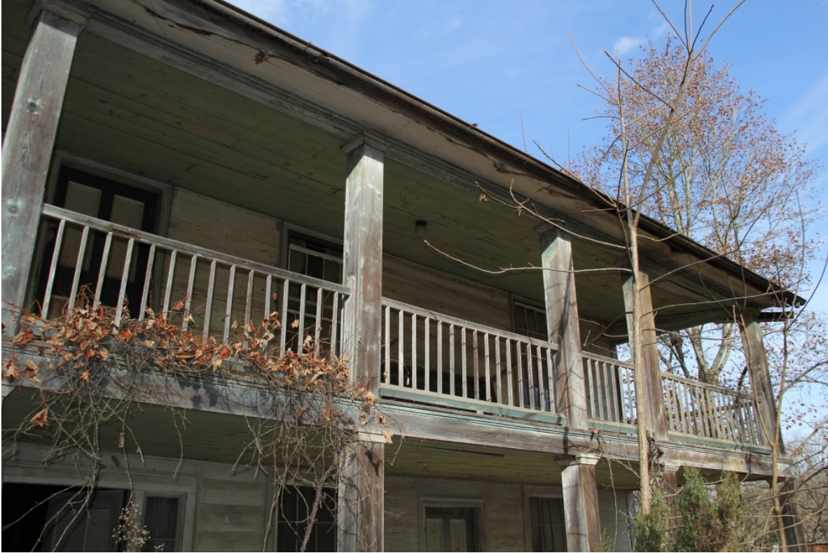
John W. Wells House, porch detail, oblique view to north
