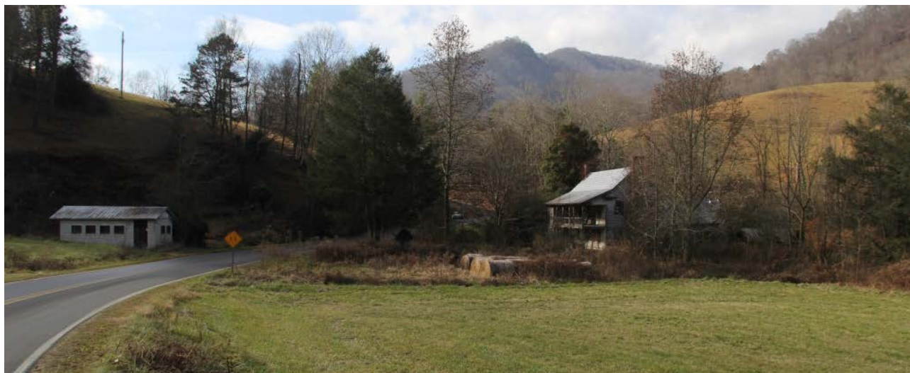
John W. Wells House (BN 749), overall view to southwest
