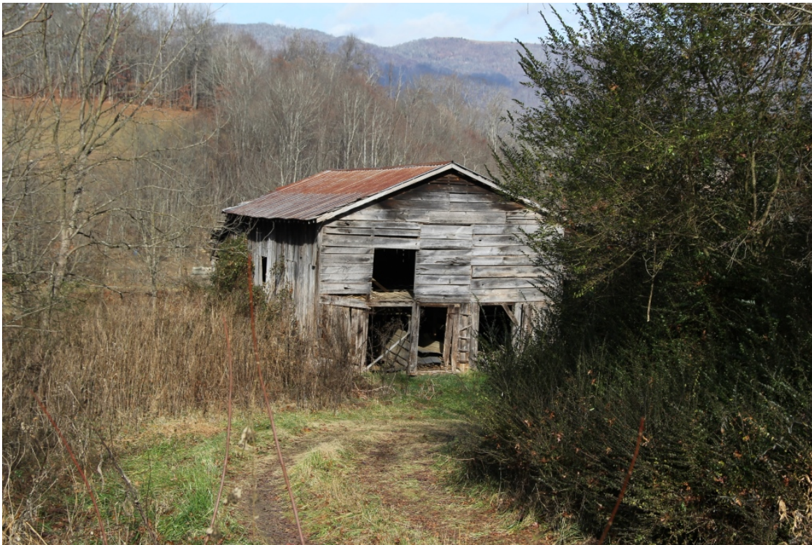
Large barn, façade, view to northwest
