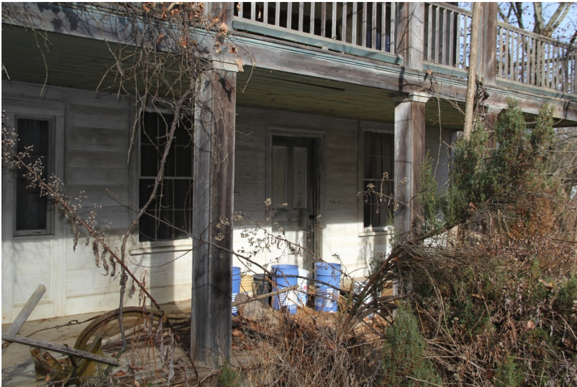
John W. Wells House, façade detail, view to north
