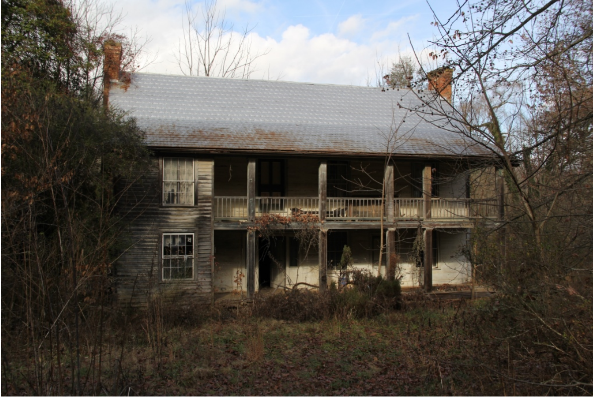
John W. Wells House, facade, view to northwest
