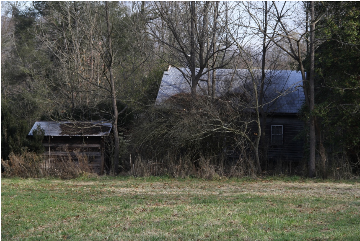
Wells House ell (r) and smokehouse (l), view to northeast
