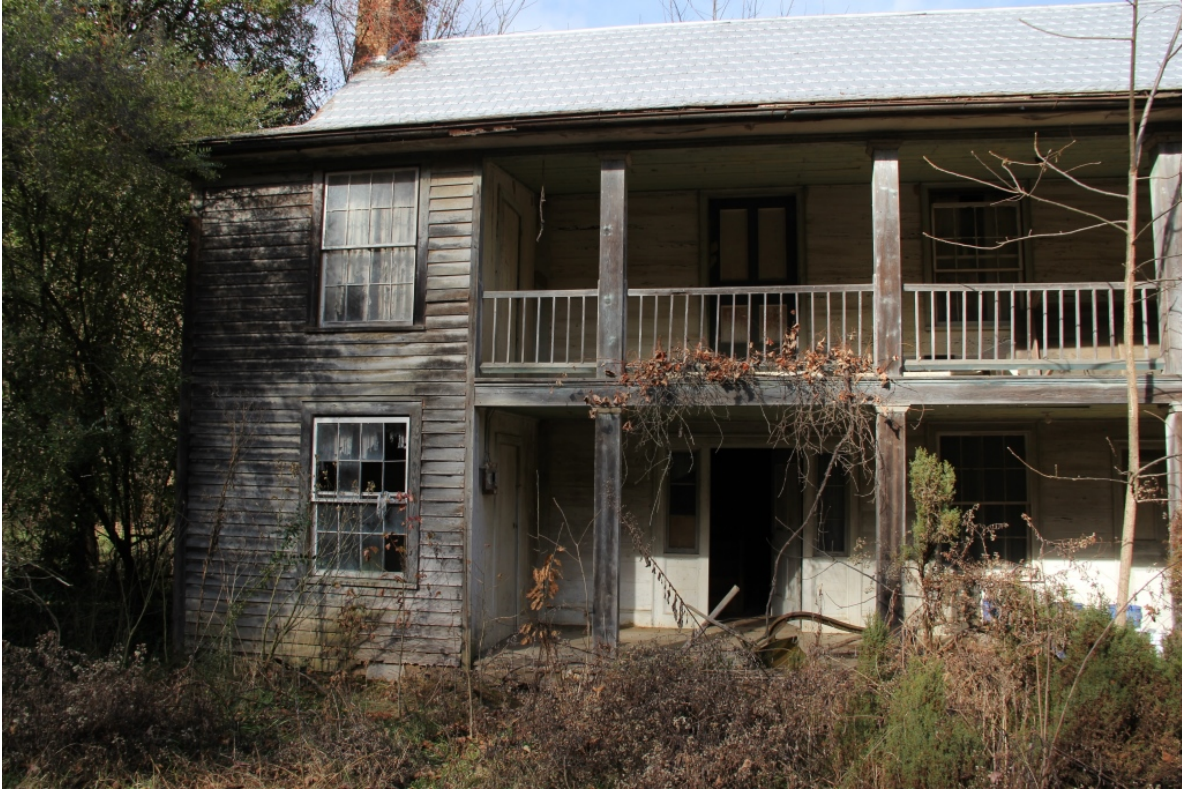
John W. Wells House, façade detail, view to west
